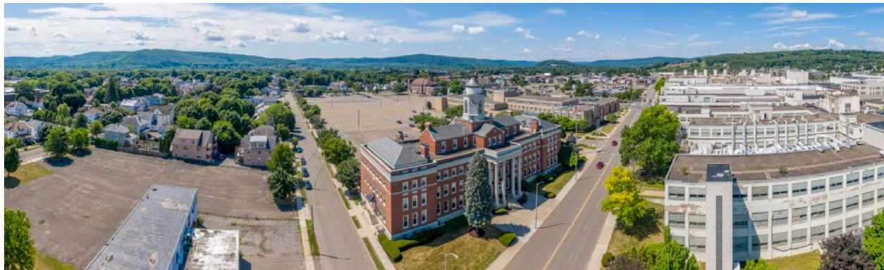
Building 32 and the old IBM buildings, before their demolition in 2025.
